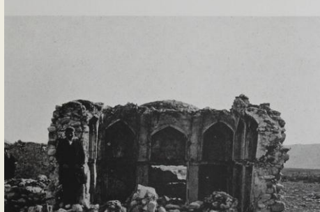
26. INTERIOR OF RUINED HOUSE AT AULISH, TĀSHĀN
